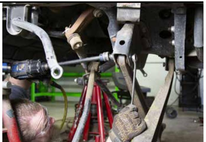
*Note: Now that the front stock suspension is off, clean the frame and prep for the radius arm bracket installation. Start by sanding down the powder coating on the radius arm brackets at the points of contact which will be welded to the frame.*
